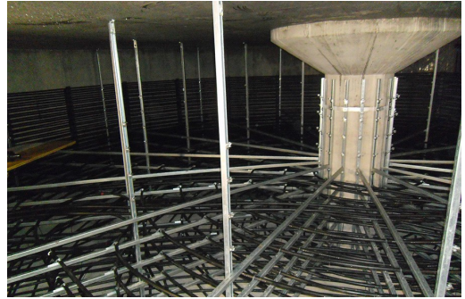
Seasonal ice storage, phase changes of freezing and melting [Kollmar et al., 2026, in preparation].
