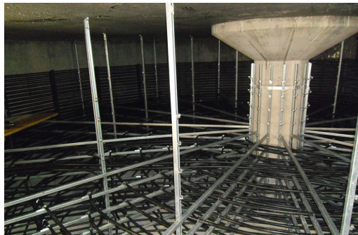
Seasonal ice storage, phase changes of freezing and melting [Kollmar et al., 2026, in preparation].
