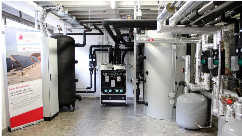
Control cabinet, cold storage, ACM, hot storage, pumps (cellar)
