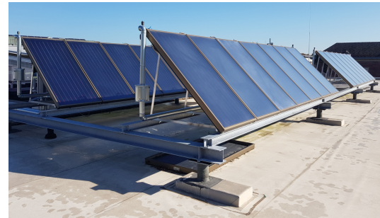
Plate collectors (roof)
