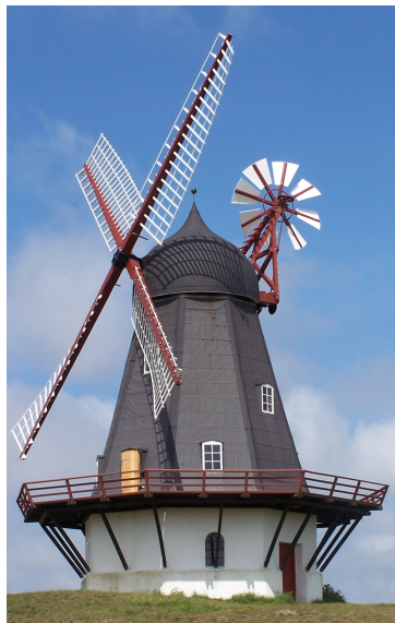
Figure 5.1: Tail-rotor used for passive control of a wind turbine.
