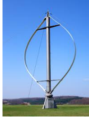
(a) Side view of a Darrieus vertical axis wind turbine.
