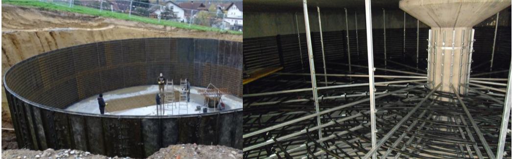
Figure: Pictures of the construction process of an ice storage 3 .
