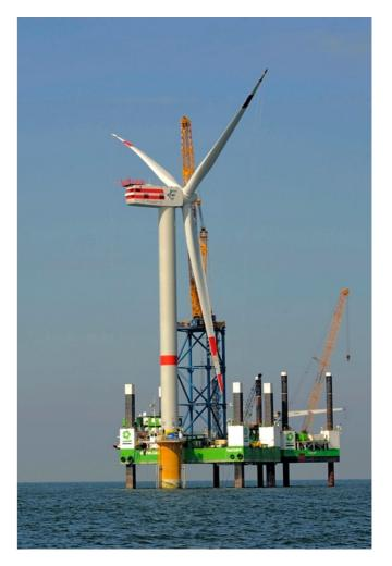
turbine and tower weigh 700 tons
