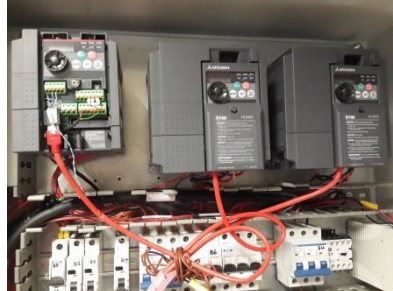
Variable Frequency Drives (VFDs)
