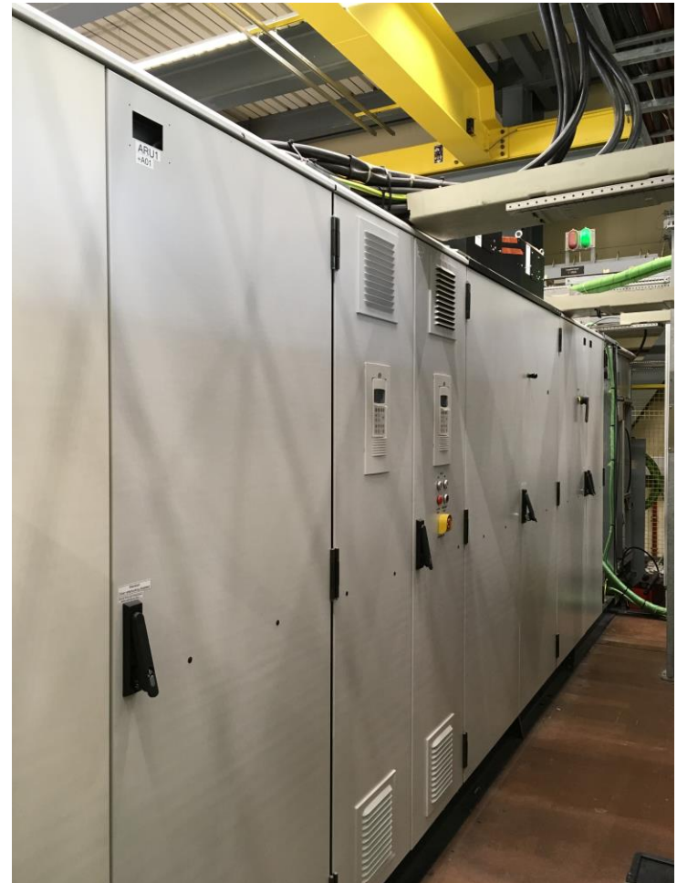
Three-level back-to-back converter:
